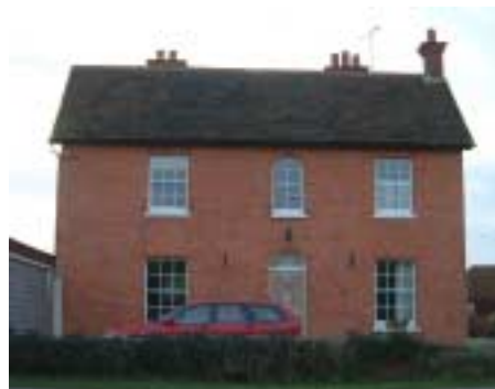
Whistley Court Farm: doors and windows well proportioned to each other, and within their elevation,
