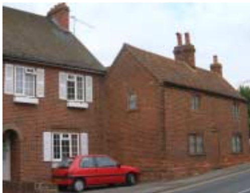
An example of white painted and stained joinery against brick elevations. The contrasting white paintwork significantly reduces the appearance of "massing", and contributes to a greater sense of spaciousness in the street scene
